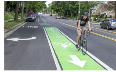
Painting bike lanes green is one way to promote awareness of the trail system's on-street facilities and improve safety.
